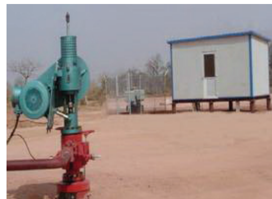
PC pump system used in oil field
